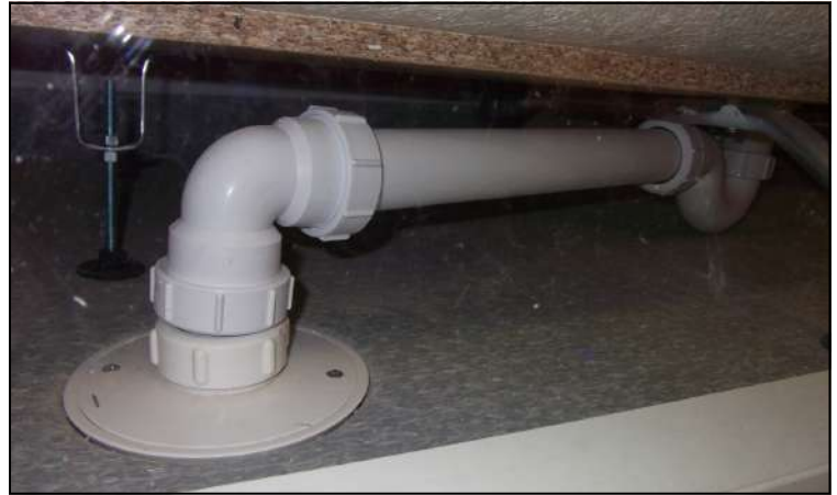
Below bath installation
