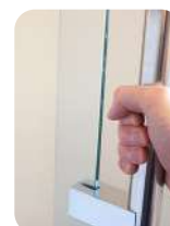
Gap between shower screen edge & grab pole: 40mm
