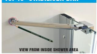
Clip the stabiliser bar onto "PANEL E"
