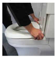
9 Complete the installation by testing the Closomat works, by again depressing the seat and holding in one of the elbow pads.
