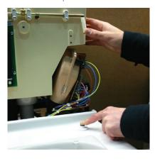
4 Should the wash splutter during the wash cycle described in step 4, the douche system may need purging to remove any potential air-lock, generated during the unit's transit/installation.
