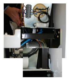
24 Push and firmly fix the soil pipe connection to the wall and Closomat. Now connect the water to your inlet and the electrics via the socket you have installed.
