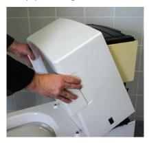
5 Correct fitted position of cistern cover clips – shown from rear of unit.
