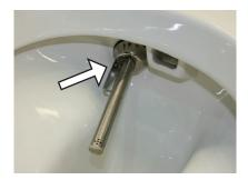
6 Should the water pressure need adjusting to suit the user, locate the pump situated on the right hand side of the Closomat. Hold down or release the pump pressure spring slide by either tightening or untightening the adjacent holding nut. Clockwise will increase the pump pressure, whereas anticlockwise will achieve the opposite.
