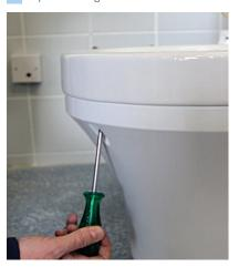
4 Replace cistern cover. Ensuring the clips on the lower rear edges engage inside the bowl cover and the on/off switch is displayed in the right hand side window.
