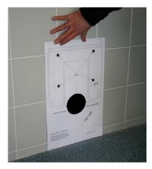
II Ensure the installation template is level.
