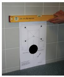
Once the installation template is secured, use to drill the wall as directed.
