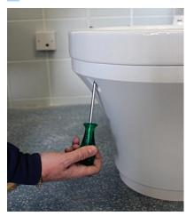
**7** Unhook the fixing adjuster brackets from the frame.
