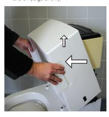
6 Loosen and remove the front screw.
