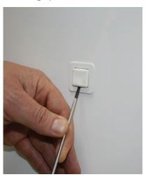
4 Loosen the screw of the cistern cover completely, but do not remove it.
