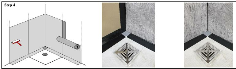
Starting from the corner carefully apply the membrane onto the wall leaving no gaps greater than 5mm between joints, at all butt joints ensure to overlap the membrane onto the joint tape by at least 70mm.
