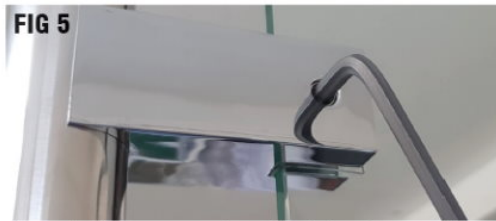
Ensure the rubber spacers are inserted in the lugs & secure to the shower screen.
